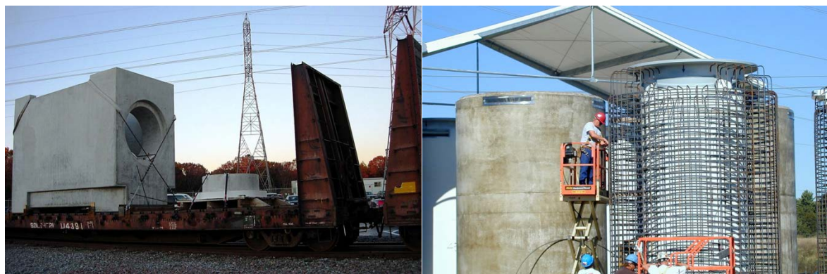
Figure 6. Horizontal storage module components in transit (left) [3]; vertical storage overpack fabrication (right) [3].
